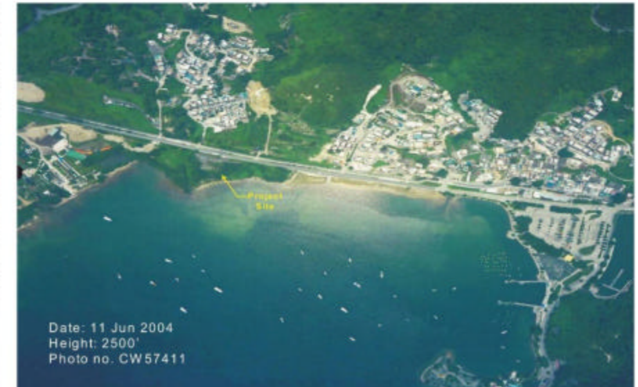
2004 - Abandoned Land with a Hard Standing Area (without any structure on top) surrounded by agriculture land and village type development
