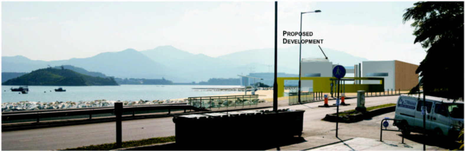
VIEW DISPLAYING THE 3D MODEL OF THE PROPOSED DEVELOPMENT DAY 1 OPERATION NO MITIGATION
