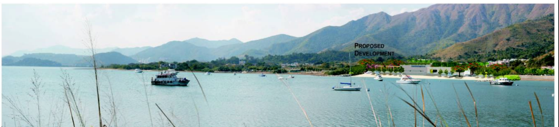
VIEW DISPLAYING THE 3D MODEL OF THE PROPOSED DEVELOPMENT YEAR 10 OPERATION WITH MITIGATION
