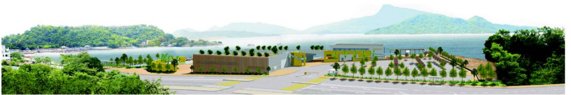
VIEW DISPLAYING THE 3D MODEL OF THE PROPOSED DEVELOPMENT DAY 1 OPERATION WITH MITIGATION
